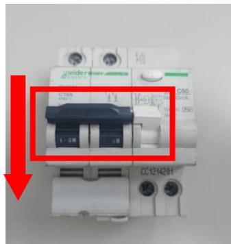
Figure 62 - AC Power Switch Off position diagram
